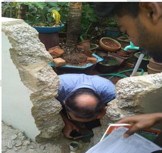
At a construction site
