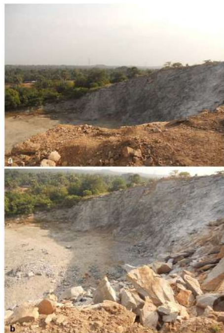
PLATE: 4 Figure a & b showing quarrying operation in progress.
